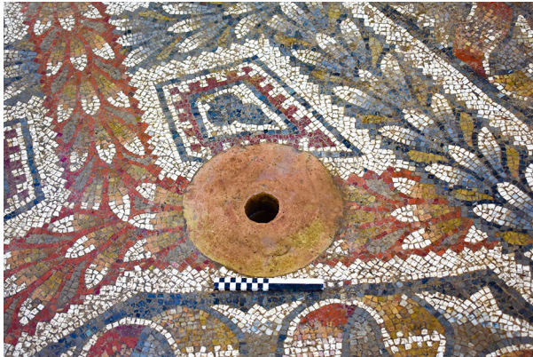
FIG. 7. Detail of the terracotta drain near the center of the mosaic floor in the frigidarium (Room 1) (scale: 20 cm).
