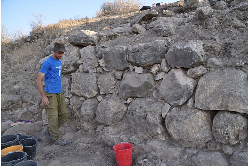
FIG. 4. The thick stone wall BB2008 on the eastern slope, with a preserved length of 11 m. Most of this building had eroded away. Floors relating to it from inside the city point to an LBA date.
